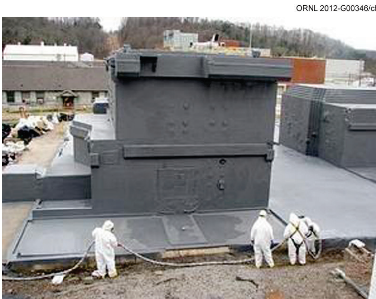
Fig. 5.42. Demolition preparations at Oak Ridge National Laboratory Building 3026 hot cells.
