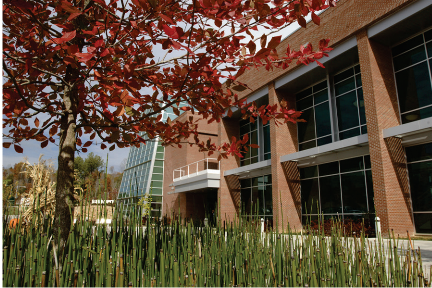
Fig. 5.10. Sustainable landscaping. [Source: Curtis Boles, ORNL photographer.]
