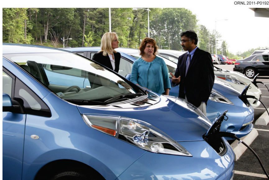
Fig. 5.9. Solar-powered charging station. [Source: Jason Richards, ORNL photographer.]
